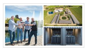
Alpha Omega says the solar power system is designed to supply nearly 100% of the winery's energy needs, and the five arrays were architecturally designed to serve as shade structures for parking and winery equipment. The new microgrid system also features Aquion Energy Inc. saltwater energy storage batteries.
